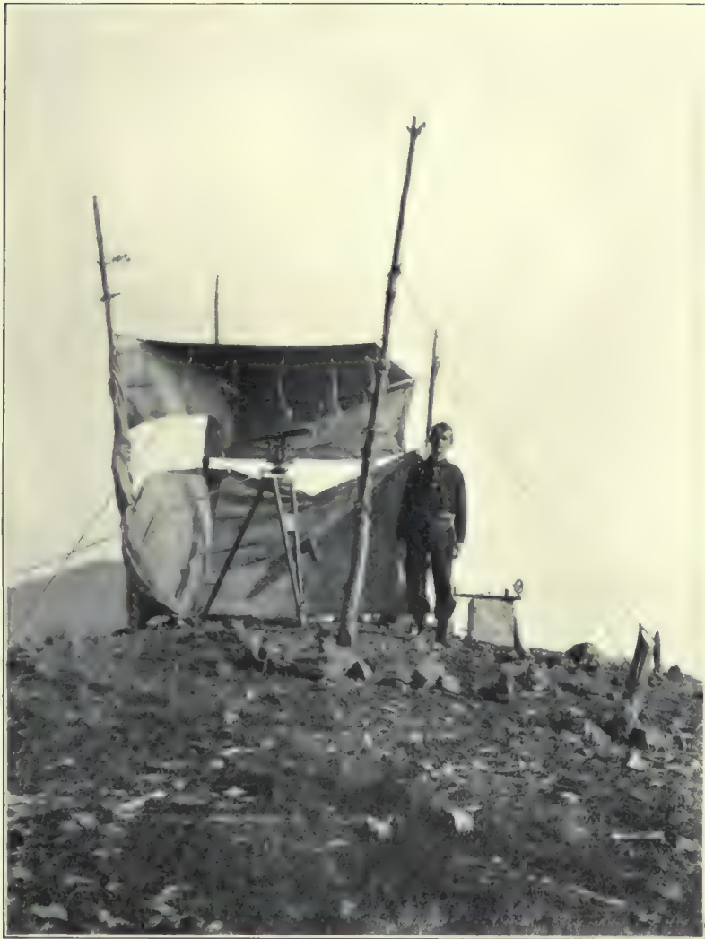
FIG. 5.—STATION BALD SHOWING THE 8-INCH POSITION INSTRUMENT IN PLACE, PROTECTED BY A WIND SHIELD.
